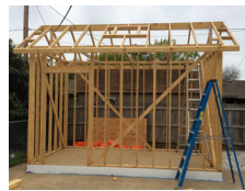
Build a Shed
