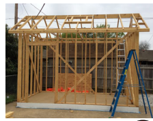
Build a Shed 21
