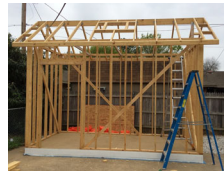
Build a Shed
