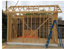
Build a Shed
