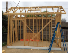
Build a Shed 21
